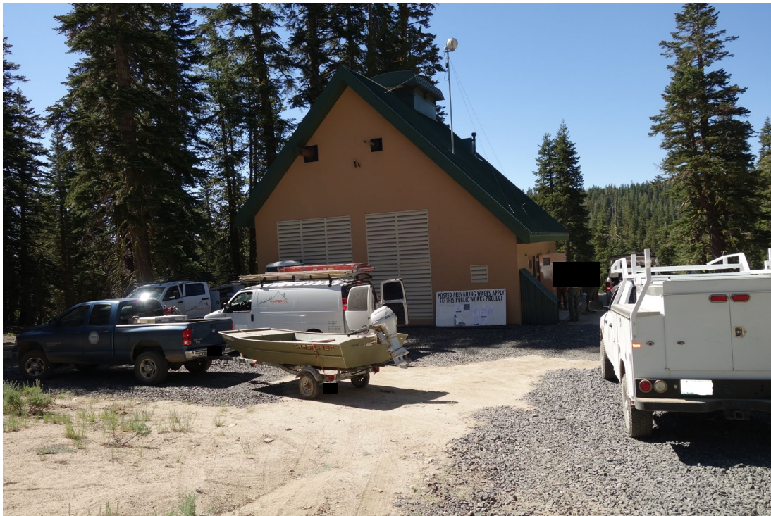
Generator Building - Building #3031 Description: View of the Building.
