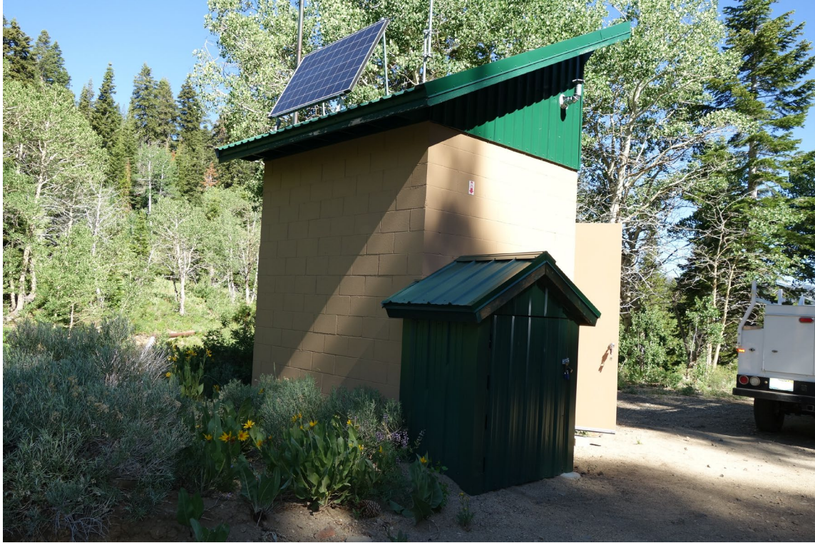
Diversion Dam Meter Building – Building #3763 Description: View of the Building.
