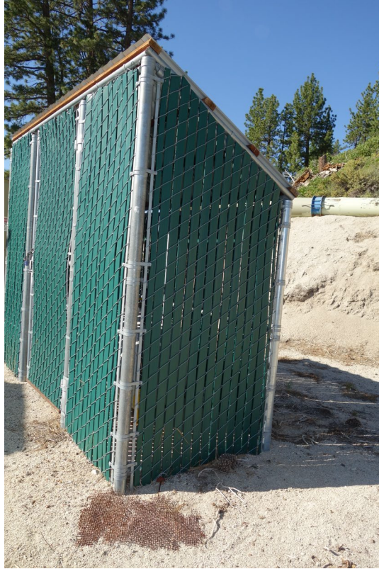
Lakeview Propane Storage Building - Building #3760 Description: View of the Structure.
