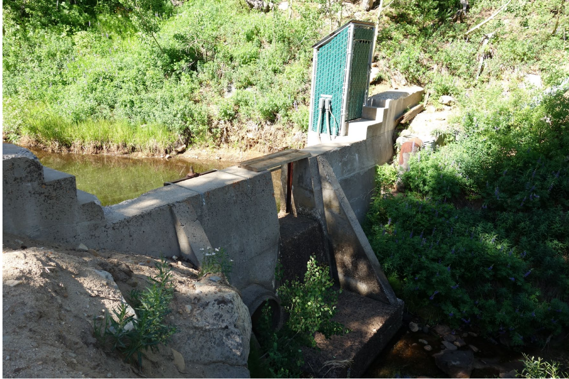
Marlette Lake Water System - Site #9788 Description: Walking Surfaces / Guardrails Needed.
