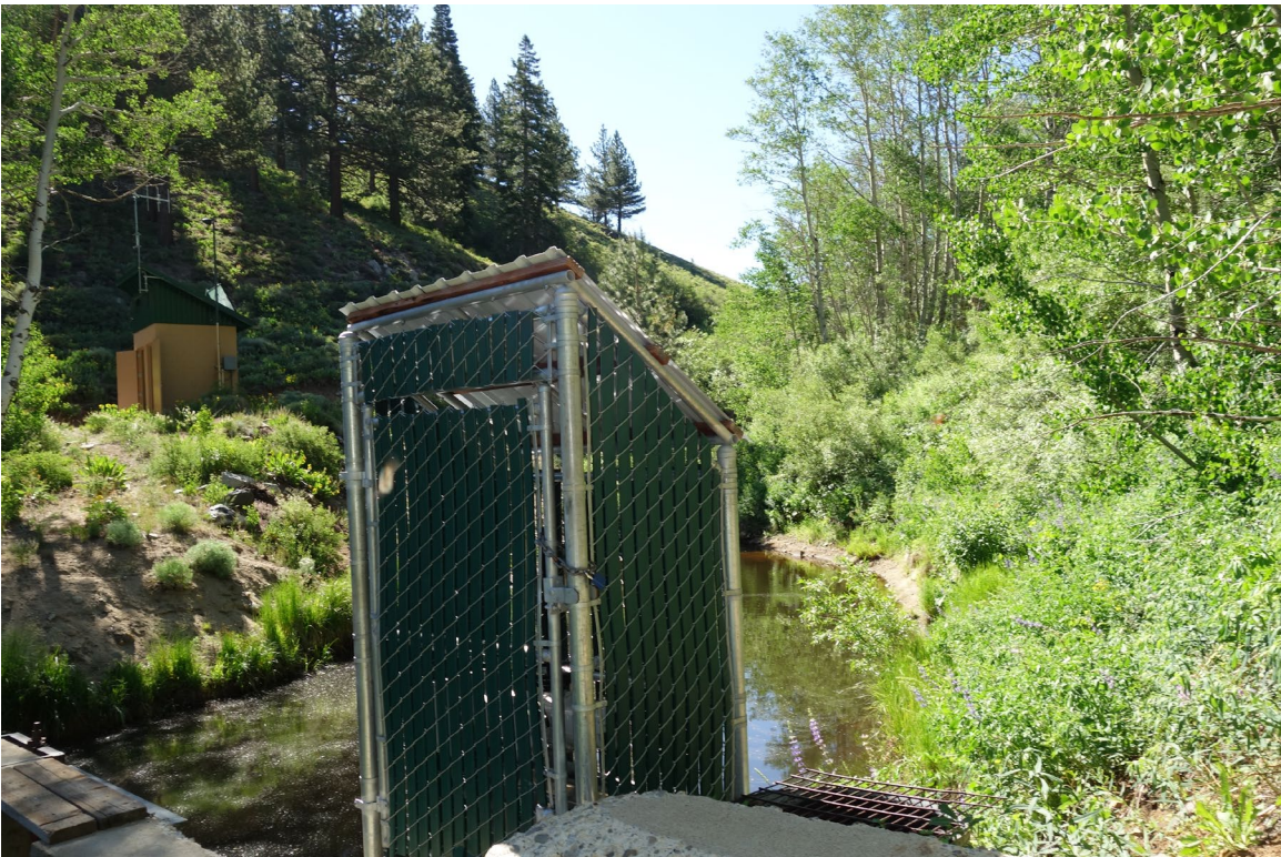
Diversion Dam Actuator Building - Building #3764 Description: View of the Structure.
