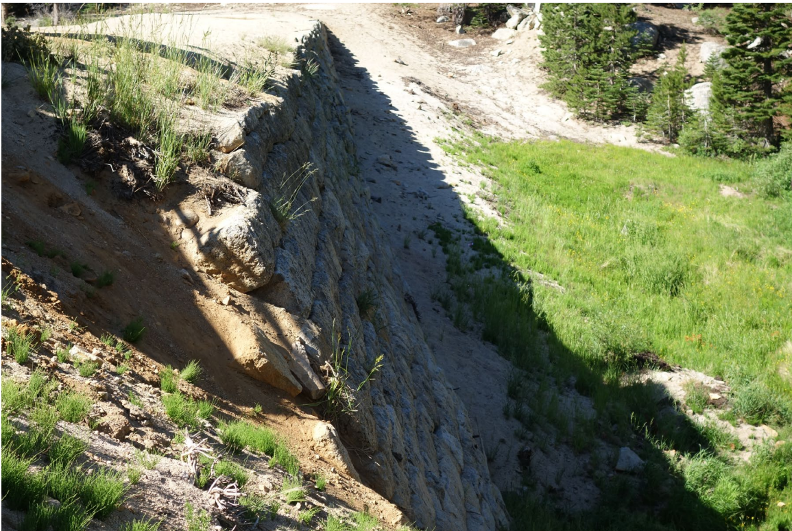
Marlette Lake Water System - Site #9788 Description: View of Hobart Dam.
