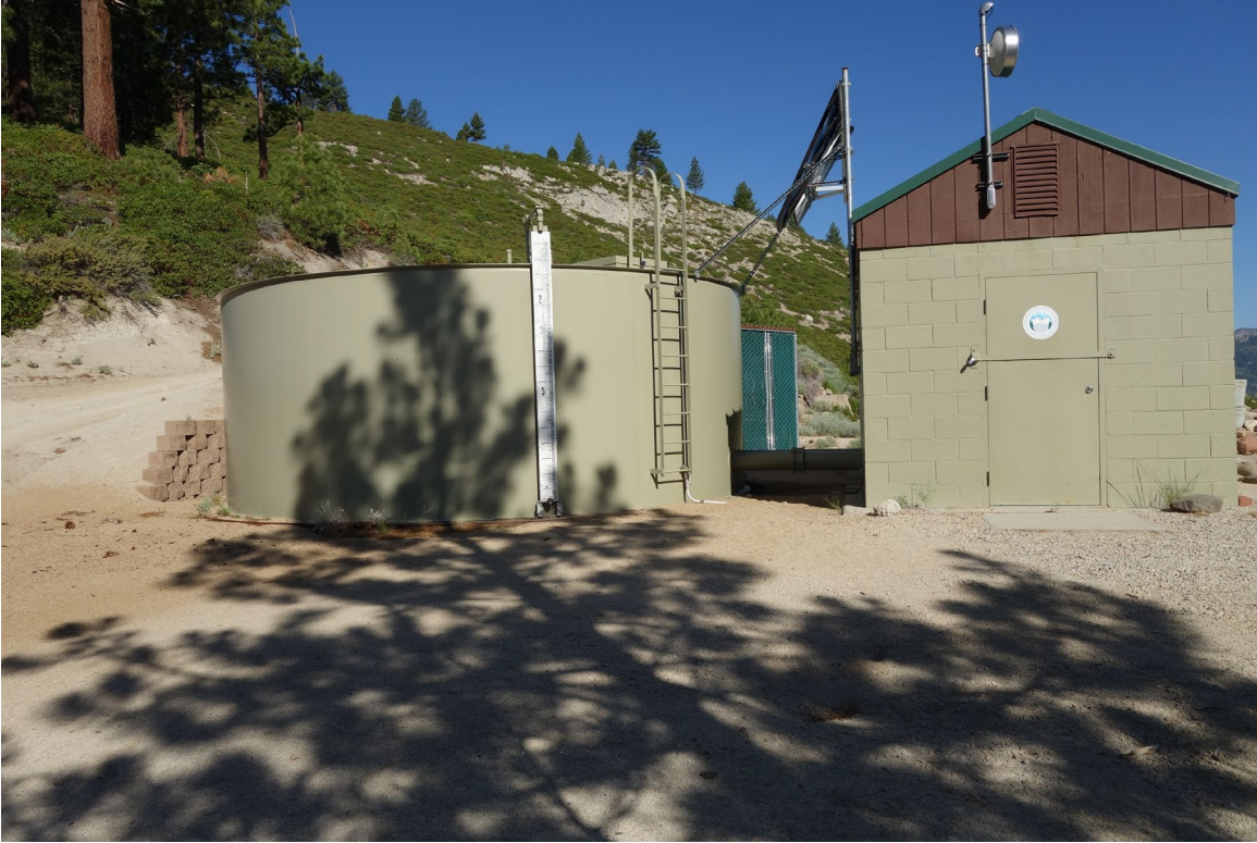
Lakeview Water Tank – Building #3762 Description: View of the Tank.
