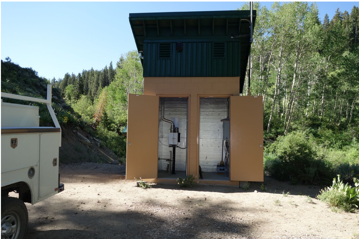
Diversion Dam Meter Building – Building #3763 Description: Exterior Landing Installation Needed.
