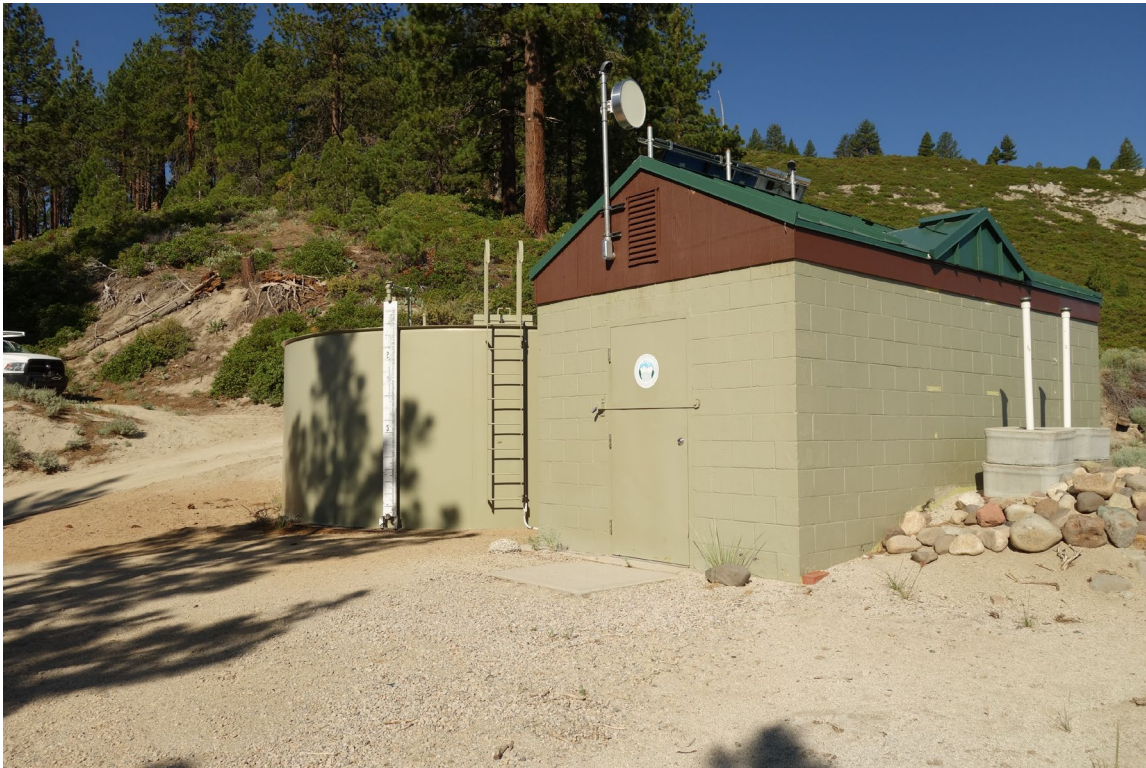
Lakeview Meter Building - Building #3761 Description: View of the Building.
